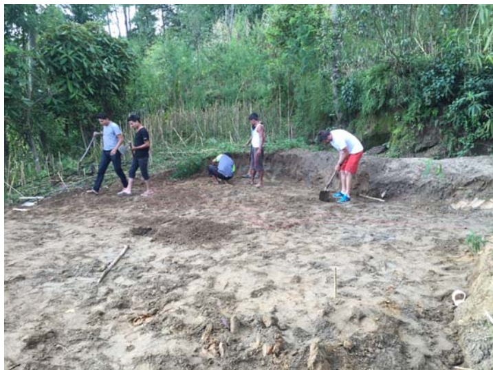
Fabrication Shop Land Clearing
