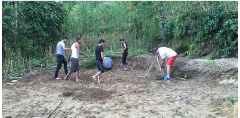
Fabrication Shop Land Clearing
